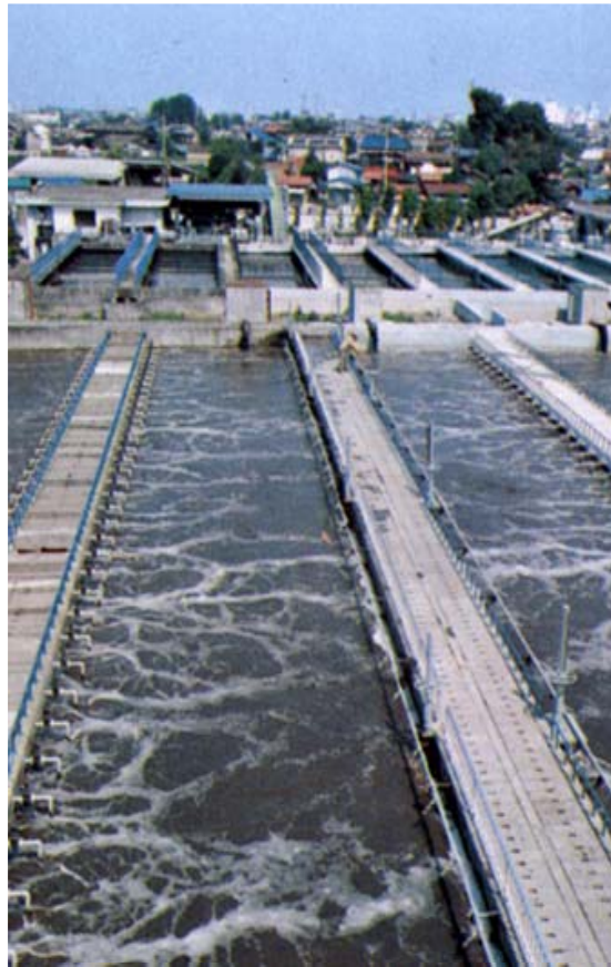
Liquid effluents treatment
